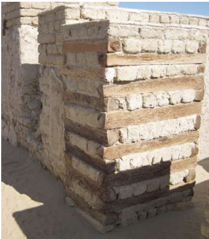
Fig. 26. Reconstructed part of a building in Medinet Maadi. Photograph by the author.
