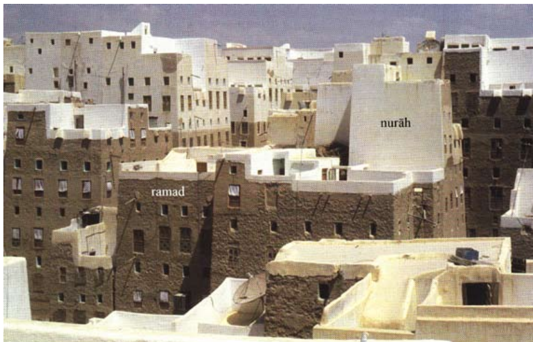
Fig. 18. Houses in Shibam showing the different types of plaster, the mud plaster ramad and the lime plaster nurāh. after Leiermann 2009, 59, fig. 69.
