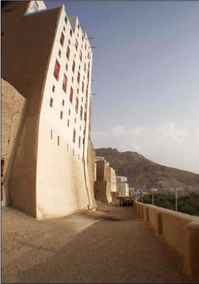
Fig. 11. Sloping outside wall of a tower house in Shibam. http://www.ilovecob.com/ashan/castles/castle24.htm .
