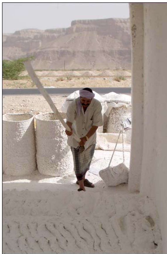
Fig. 20. The beating of the lime powder until it becomes nurāh plaster. http://ilovecob.com/ashan/mudmasters/mm18.htm .
