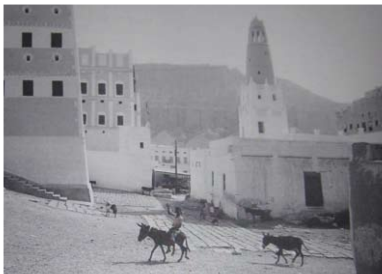
Fig. 30. Drying bricks in the streets of Shibam. Damluji 1992, 87, 3rd picture from top.
