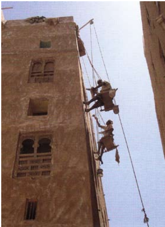
Fig. 31 Renewing of the façade of a tower house in Shibam. Leiermann 2009, 79, fig. 97.
