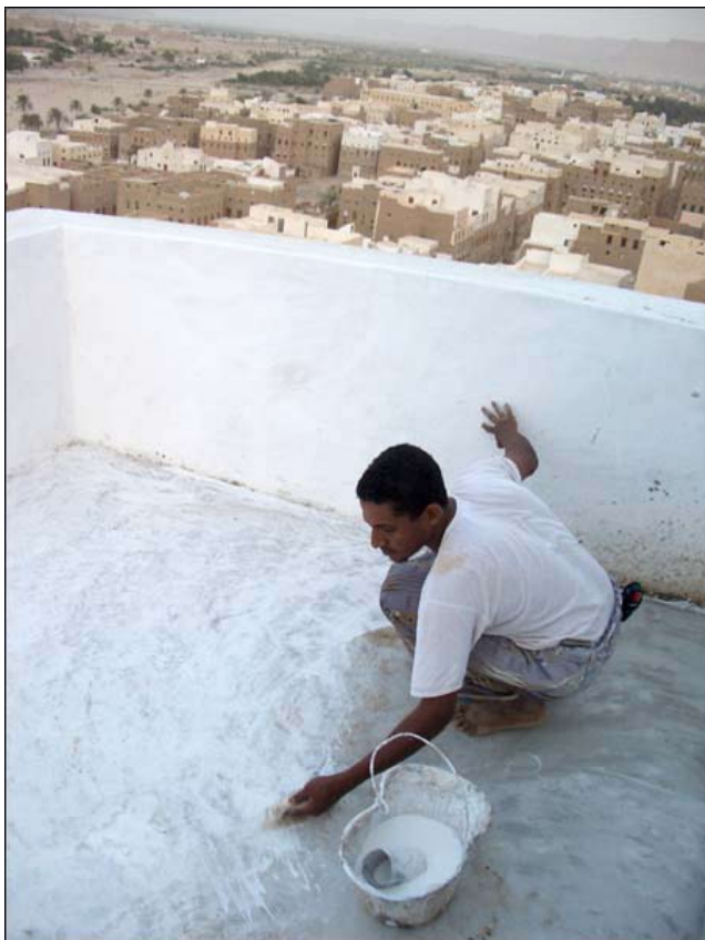
Fig. 21. Nurāh plaster being applied on a roof in Shibam. http://ilovecob.com/ashan/mudmasters/mm30.htm .
