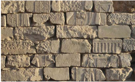
Aswan (Syene). Blocks of the temple of Tiberius, reused in the town wall. Photograph © Swiss Institute for Architectural and Archaeological Research, Cairo
